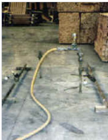
Figure E-8: Illustration of Pressure Grouting
