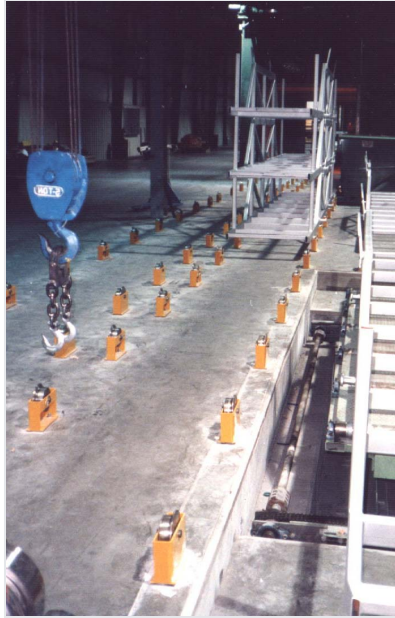
Figure C-28: Floor-mounted conveyor rollers for baskets
