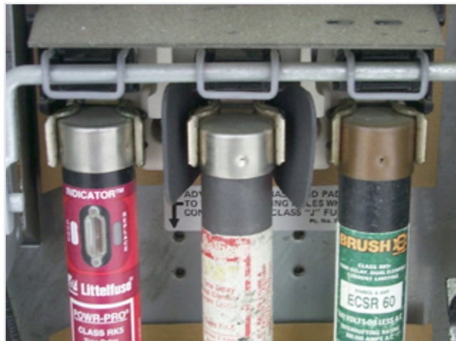
Figure 6-7: Overheated fuse block identified by infrared scan.
