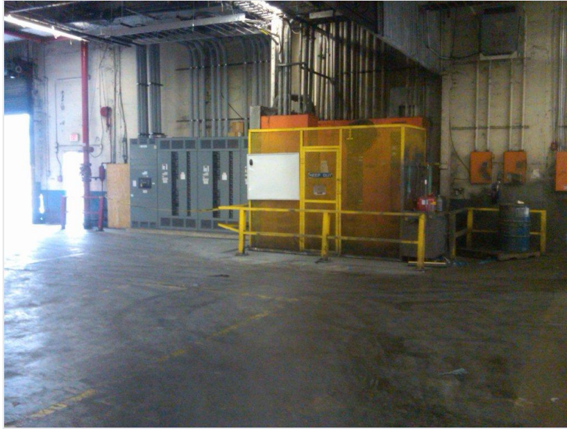
Unprotected Switchgear
