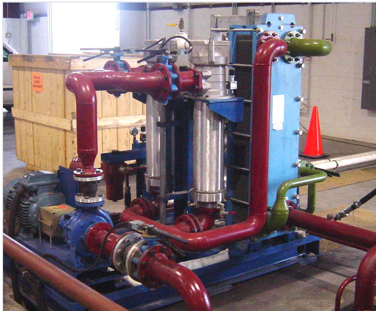
Figure 5-2: Filtration by "kidney loop"
