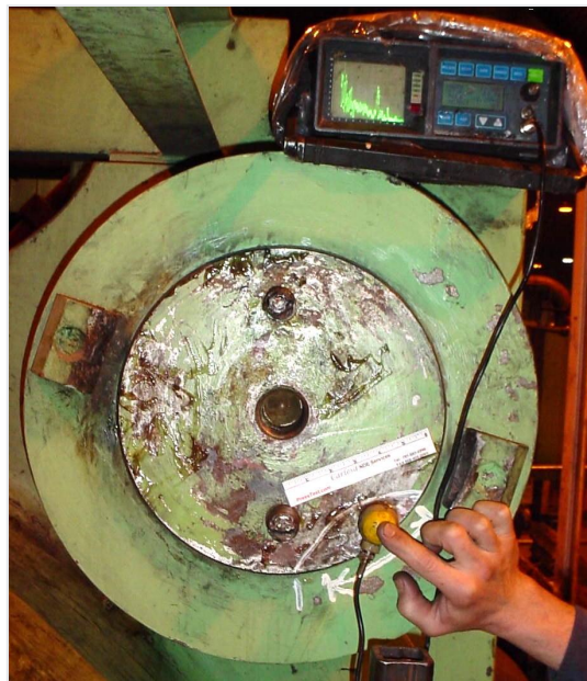
Ultrasonic indication of a tie-rod crack
