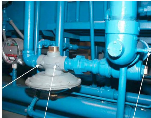
Figure 7-12: Adjustment of fuel gas supply pressure (Photo courtesy of Belco)
