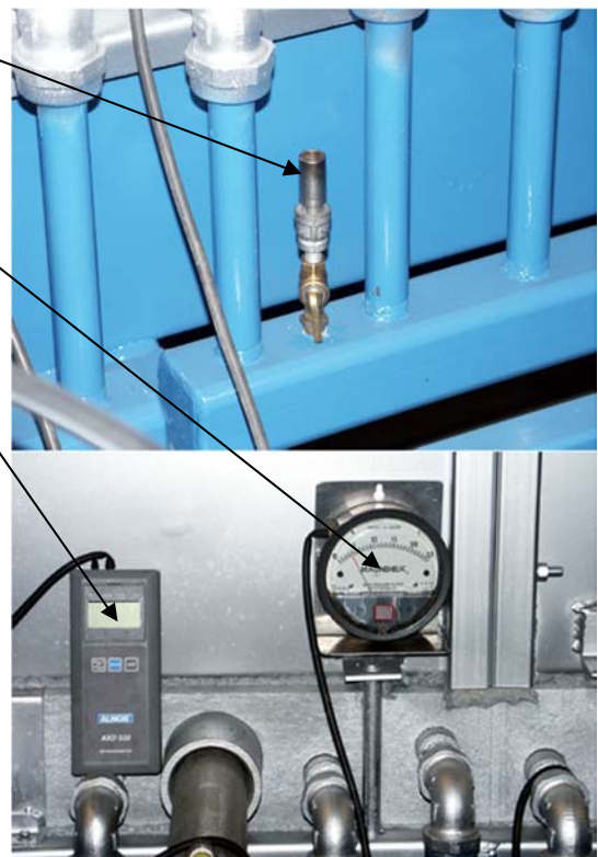
Figure 7-11: Tools for combustion setup (Photo courtesy of Belco)
