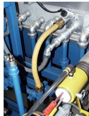
Figure 7-13: Pilot burner and flame detector (Photo courtesy of Belco)
